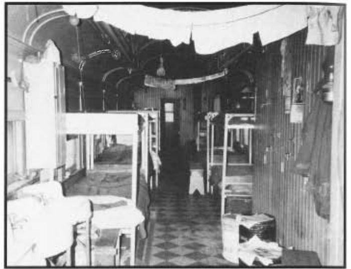
Interior view, SLSF 102743 Bunk Car Frisco photo
