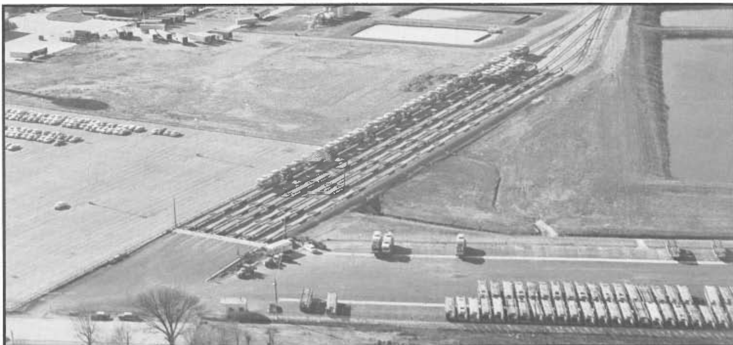
Frisco's automobile facility at Valley Park (St. Louis) showing loading tracks with capacity of 50 tri-level or bi-level cars and adjoining storage area. Frisco photo
