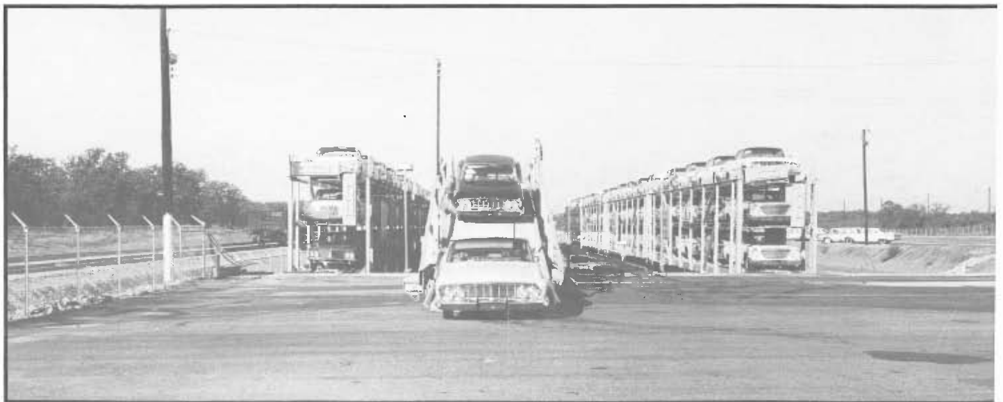
Frisco's Irving, TX automobile ramp showing Buck Unloader.
