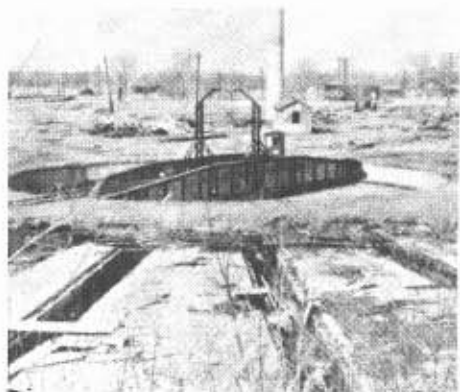
When the backshops caught fire on July 22, 1957, the wooden stalls were destroyed and the brick portion was gutted.
