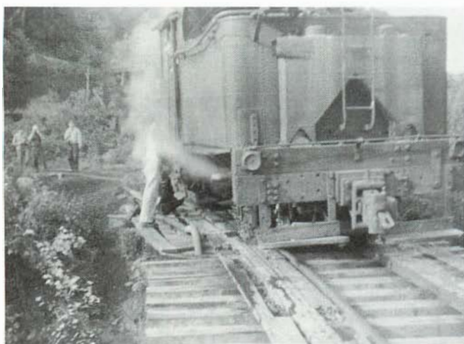
Shay #8 taking on water from the creek at Clifftop. Note that link-and-pin coupler is still being used. May 1955.
