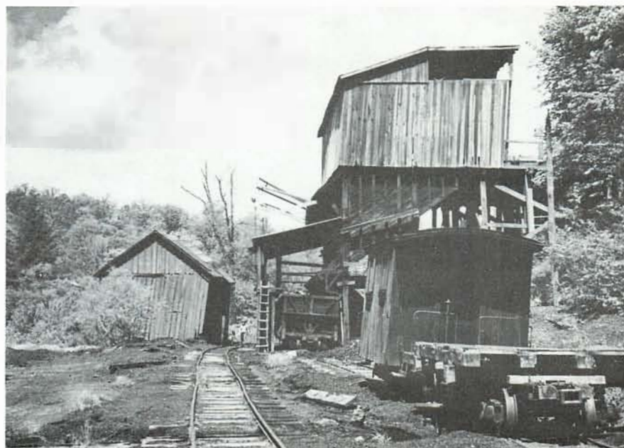
Strip tippie at Clifftop, circa 1950, near the end of operations. Last caboose is at right with flatcar. Note hopper spotted under tippie, and operating levers and cables. Track-age to Mine #10 snakes between tippie and dilapidated shed.
