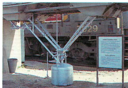
Pipe and tank detail — originally gray, it is now silver. March 1991.
