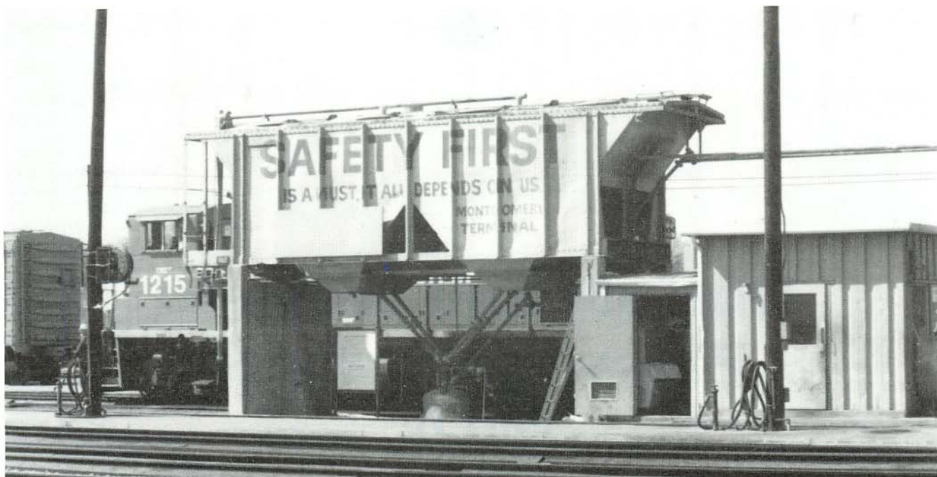
The CSX sand storage tower.
