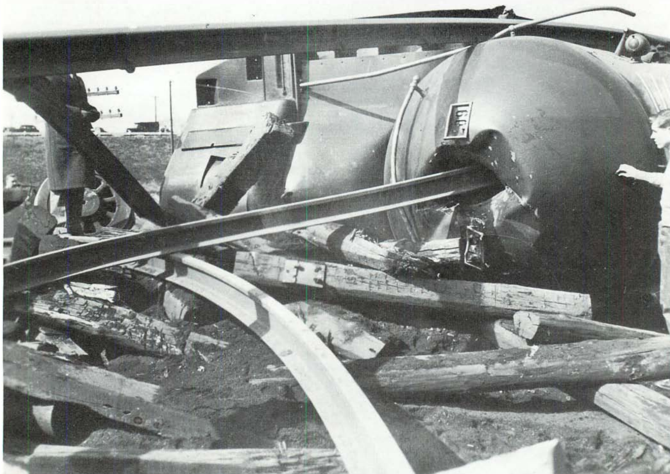
A rail pierces the nose of Class J No. 607 after it left the rails at nearly 80 mph. The spoked wheel to the left is one of the engine's pony-truck wheels which normally guided a steam engine into curves. Photo is believed to be of the February 20, 1948, wreck at Franklin Furnace.
